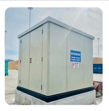
The system of a transformer station and low voltage cabinet, including 01 Incoming Circuit Breaker 1250A and 03 Circuit Breaker 300 A.
